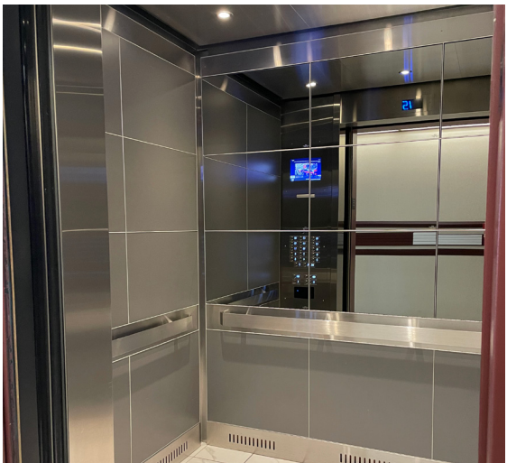
Complete elevator cab retrofit with flush mounted LED screens
